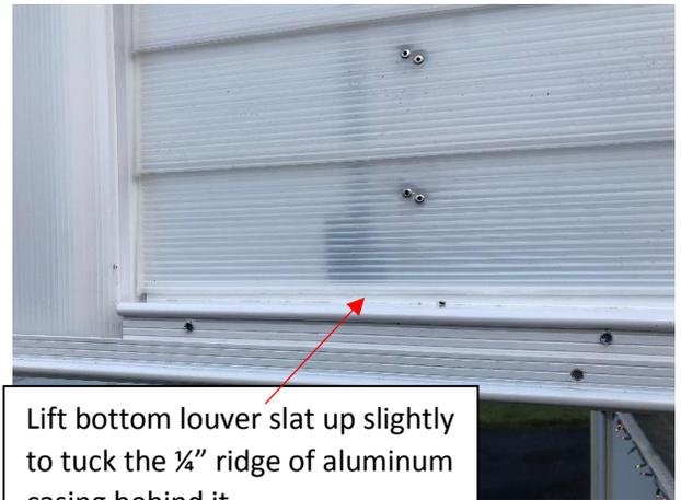
Lift bottom louver slat up slightly to tuck the 1/4" ridge of aluminum casing behind it
