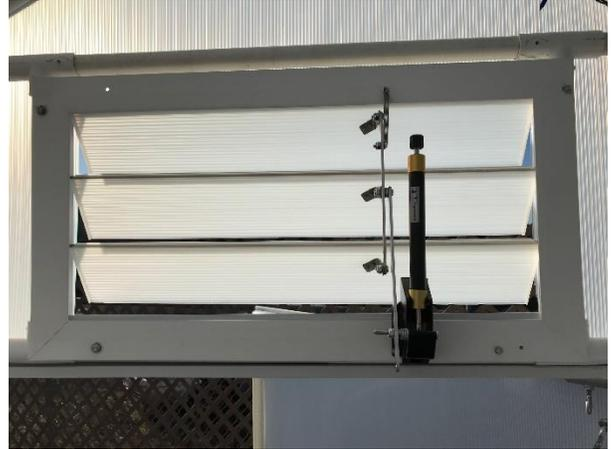
9. From outside the greenhouse, slide the 22 3/4" Aluminum Casing over the bottom of the louver frame (you will need to slightly lift up the bottom louver slat). Line up the Casing holes with holes in the Louver and attach with 1" Screws.
